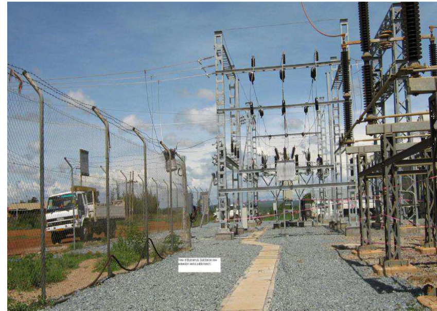
10MVA 220/33kV Bulyanhulu Substation, a view of 33kV Bus for Kahama Shinyanga Water Supply Project -Ministry of Water December 2007
