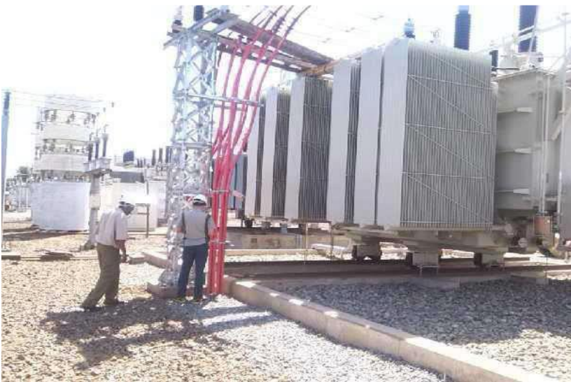
50MVA, 132/33kV Transformer at switchyard with Connected Power Cables.
