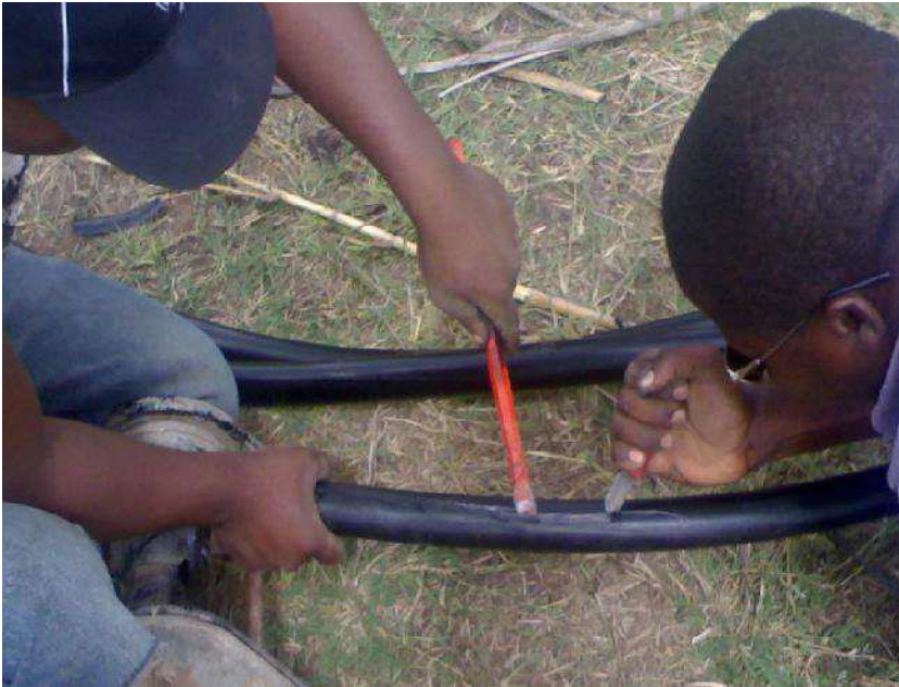
Removal of PVC cover of 33kV, 95mm 2 marine cable as preparation for cold termination for Kahama Shinyanga water supply project -Ministry of Water October 2007
