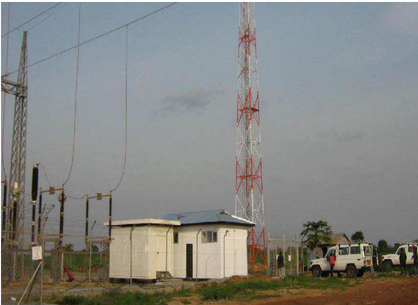
A view of a new constructed 10MVA, 220/33kV Bulyanhulu Substation showing a new erected 30metres Communication Tower for Kahama Shinyanga Water Supply Project - Ministry of Water December 2007
