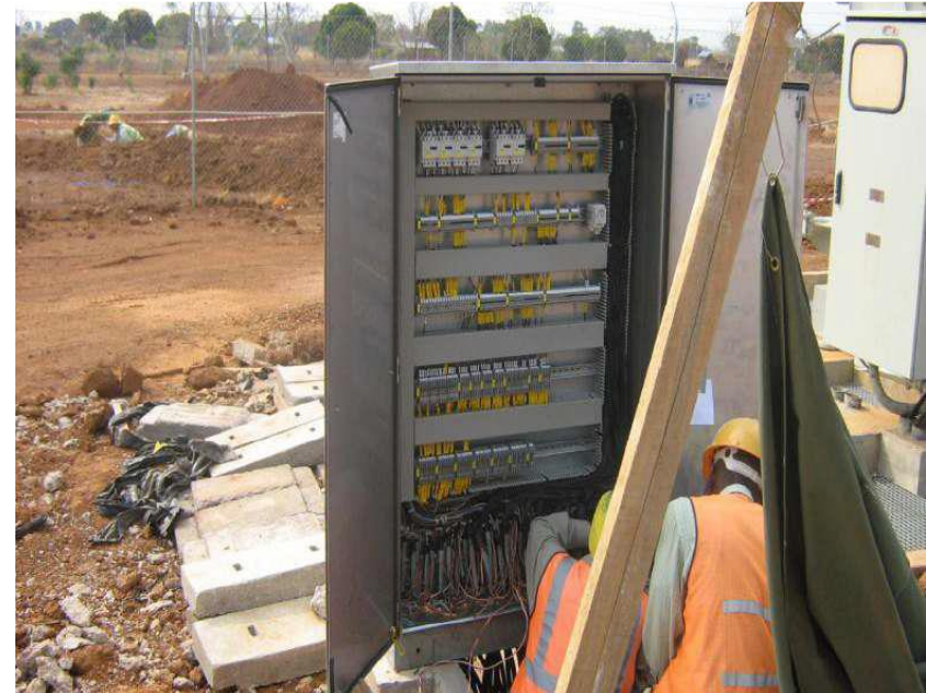
Technicians conducting wiring at control panels and marshalling panel at Buzwagi Gold mine project October 2008
