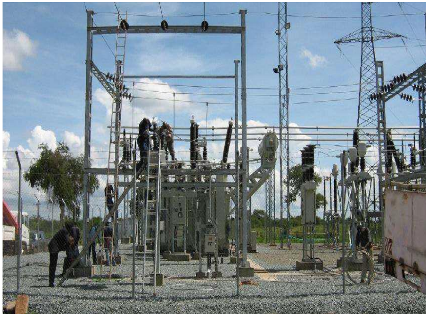
Erection of one-unit 10MVA, 220/33kV Transformer for a extended bus for Bulyanhulu Substation for Kahama Shinyanga Water Supply Project -Ministry of Water December 2007
