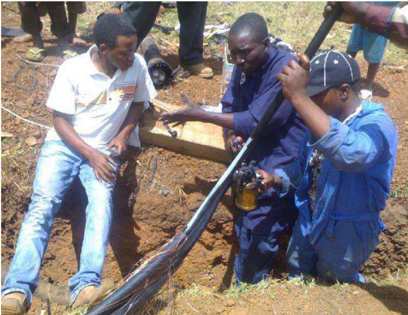
Cold termination for the 33kV, 95mm 2 marine cable across Lake Victoria-for Kahama Shinyanga water supply project - Ministry of Water October 2007
