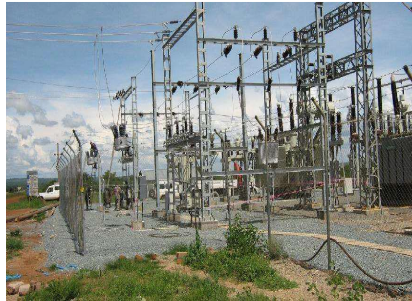
A view of a new constructed 10MVA, 220/33kV Bulyanhulu Substation for Kahama Shinyanga Water Supply Project - Ministry of Water December 2007
