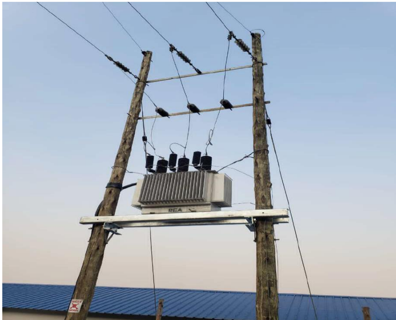
MFE Installation works of distribution transformers at Hoima EACPO pipeline oil drilling Stations-Uganda
