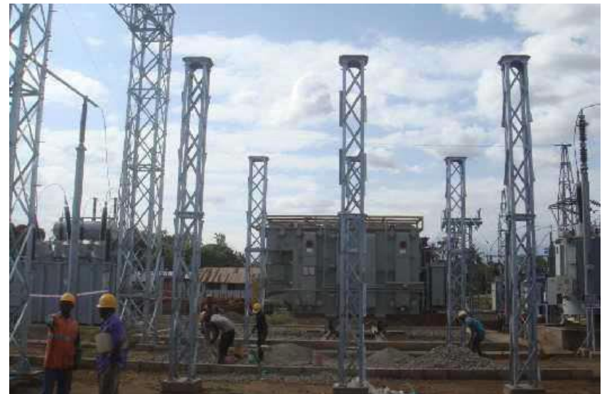
Switchyard Structures completed ready for Equipments Installations.
