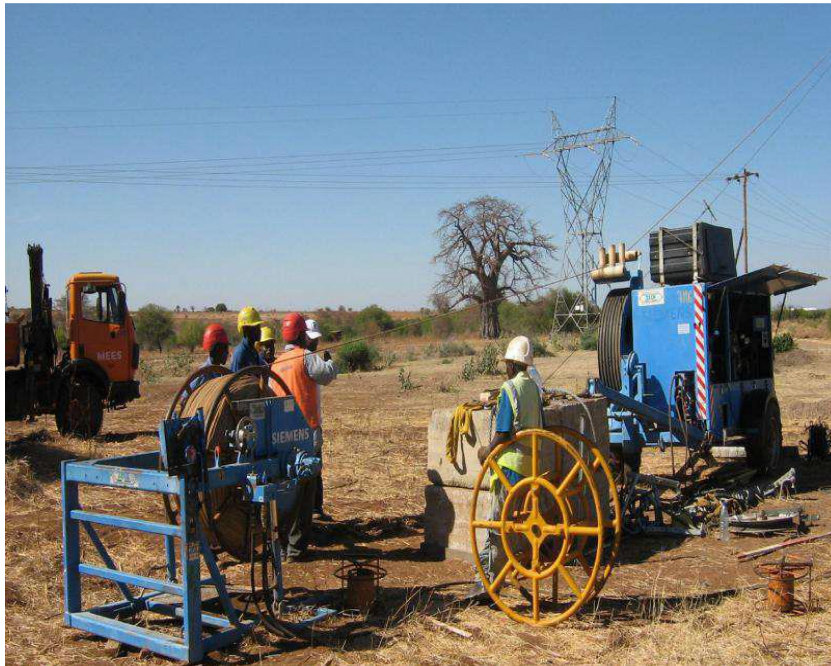
Construction of a 220kV power line, picture showing our linesmen with Conductor/cable Winches with jacks for stringing works for Shinyanga – Buzwagi 220kV Powerline- September 2008
