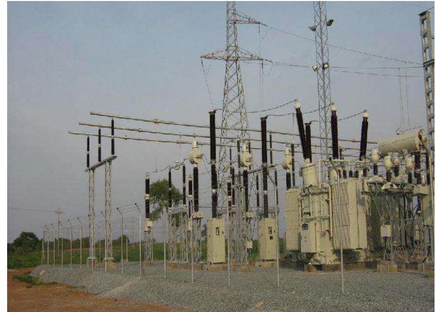
A section view of a new constructed 10MVA, 220/33kV Bulyanhulu Substation showing an extended 220kV Bus, and other switch gears for Kahama Shinyanga Water Supply Project -Ministry of Water December 2007
