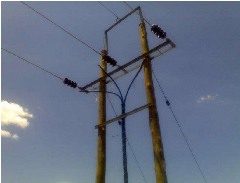
A view of a new constructed 33kV Overhead Power line at H terminal Pole structure point where a 33kV, 1.8km marine cable was terminated at intake point before crossing Lake Victoria, at Nyamtukuza Village- Geita District – Mwanza for Kahama Shinyanga Water Supply Project for Ministry of Water - December 2007
